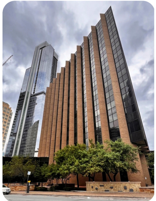
Charles' interest in architecture drew him to taking this photo of the Travis County Offices at 700 Lavaca
